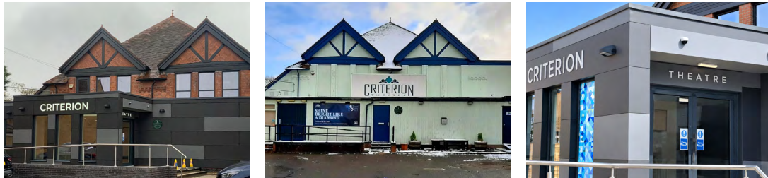
How building work has transformed the exterior of the Criterion from 2021 to 2025. Photographer: Anne-marie Greene.
